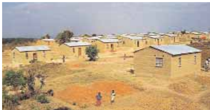
Houses by Habitat. No, not that Habitat
